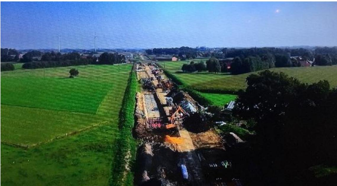
Picture 1. Conventional installation of cables in open-trench, Raesfeld, Germany
